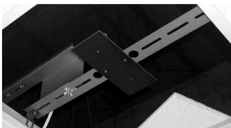
UFODAP1200 installed above ceiling
